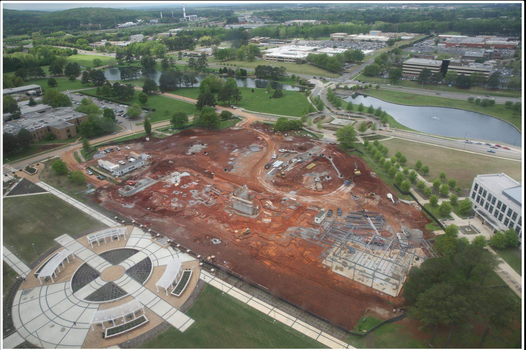
Student Services Building Construction
