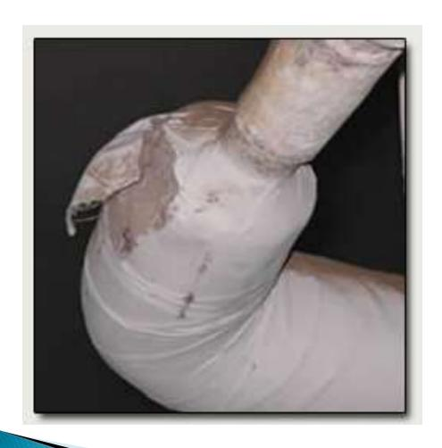
Asbestos pipe and boiler insulation does not present a hazard unless the protective canvas covering is cut or damaged in such a way that the asbestos underneath is actually exposed to the air.
