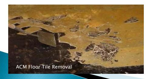
Asbestos is most hazardous when it is friable. The term "friable" means that the asbestos is easily crumbled by hand, releasing fibers into the air. Sprayed on asbestos insulation is highly friable. Asbestos floor tile is not.
