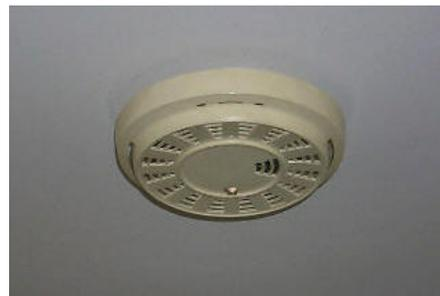
A better alternative to battery-operated devices is “hard-wired” single-station smoke alarms. These devices receive their primary power from a 120-volt electrical circuit in the building. This arrangement is typically required in new buildings, where it is a relatively simple matter to provide electric power to the smoke alarms. The Hotel and Motel Fire Safety Act of
