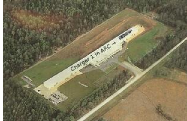
Figure 12. Aerophysics Research Center, the building housing Charger 1.
