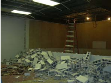
Knocking out the wall between classrooms 405 & 406
