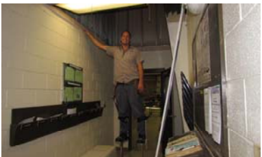
Allen replacing PPB ceiling grids
