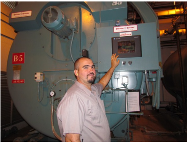
Josh at Central Plant
