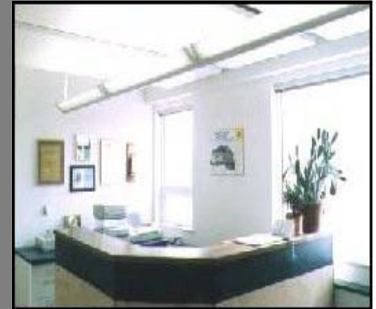
Indirect lighting reflects most of the light off the ceiling.
