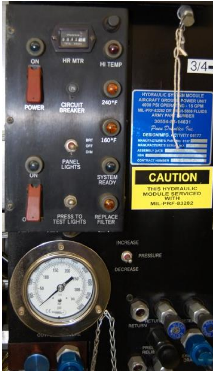
Figure 4: Current Hydraulic Module Control Panel
